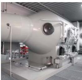
Extract air is drawn directly from the space above the baths and scrubbed before being exhausted. Heat energy is recovered and recycled.
